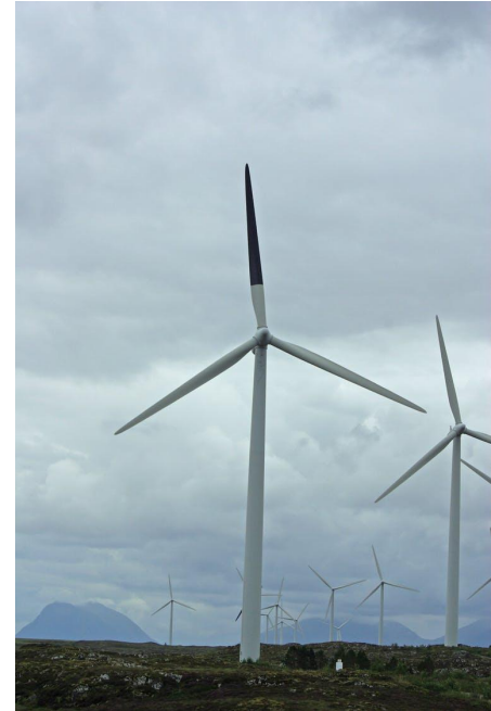
One of three blades was painted black on the four study experimental turbines, which was thought to help birds see the whirling blades more easily. From Ecology and Evolution journal under a Creative Commons license.
